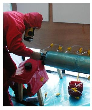
asbestos, and know that it does not take up wetting agents uniformly. If there is leakage at an injection point the System can respond instantly by slowing down or even stopping delivery of the wetting fluid at that point, so there is no messy spillage to clear up.
